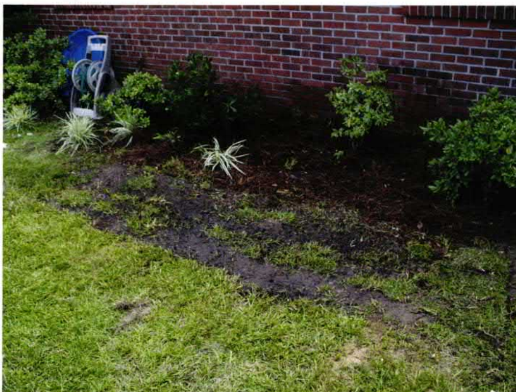
Picture 2: UST 1277Flamingo excavation site after completion of work.
